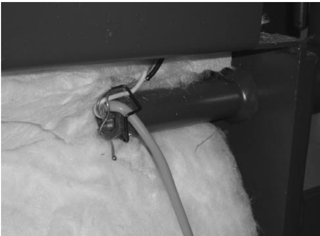
Fig. 15 – View of the water temperature sensor TK in the boiler pocket - boiler with burner in the top door - DCxxS(X), CxxS, ACxxS, DCxxRS
