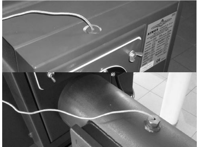
Fig. 14 – View of the flue gas sensor TS or TSV in the flue gas duct pocket. For boilers D30P and D45P is placed on the flue gas channel
